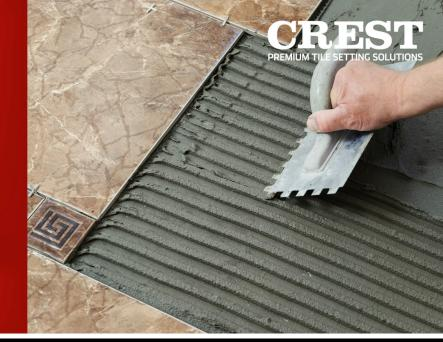
CREST PLATA® is a fortified and non-modified thin set mortar, specially designed for the installation of ceramic tiles with high and medium water absorption such as ceramic, quarry or Saltillo tiles. For floors and walls, indoor use. Ideal for residential and commercial use.
