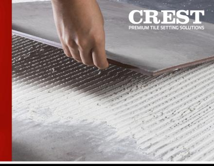
CREST GRAN FORMATO® is a polymer fortified large and heavy bed mortar formulated for the installation of large size porcelain and ceramic tile, marble, granite and natural stone. Specially designed for solving shrinkage problems. Contains a specific particle size of sand that improves the stability and enhances the slump resistance.
